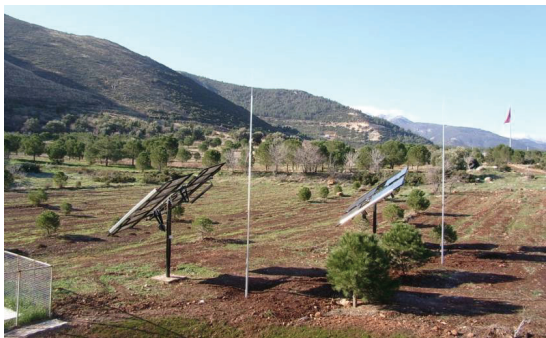
Fig. 4. CEH with air termination rods
