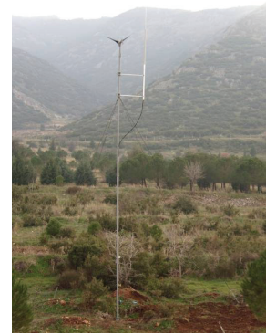
Fig. 6. Wind turbine with HVI air termination rod
