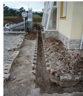
Fig. 3. Digging work for the round grounding
