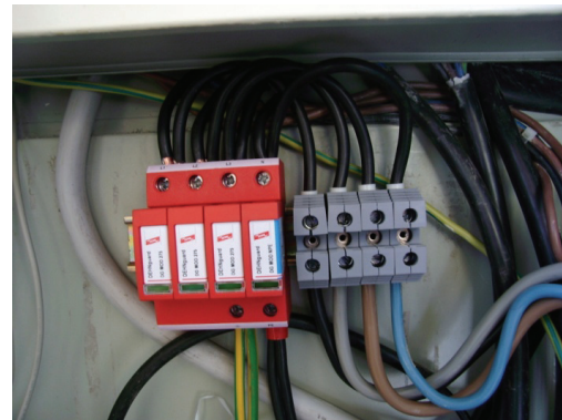
Fig. 7. 3-phase surge arrester
