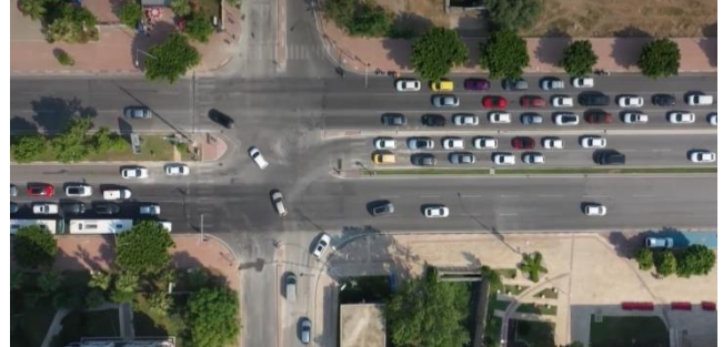
Fig. 1. Antalya Heybe intersection structure.
